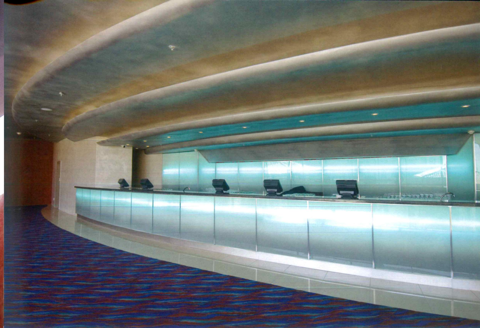
The bars on the Rear Stalls Level are recessed under the auditorium's raked seating.
